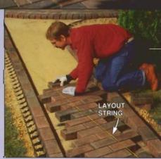
LAY THE PAVERS using a string for a guideline. Cut and install pieces that butt up to the border later.
