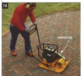
TAMP THE PATIO with a flat-plate vibrator after all the pavers are installed. Tamp entire outside edge first, then circle in.
