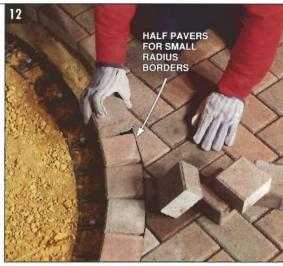
USE HALF PAVERS for bordering tight circles. Smaller pavers cut down on the size of the pie-shaped gaps between each piece.
