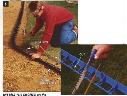
tamped subbase using 8" - 10" spikes. Cut the webbing on the edging's back side to make it flex for curves.
