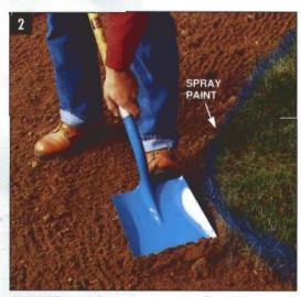
REMOVE SOD in an area extending 8 in. beyond the boundaries of the patio. Spray paint indicates the excavation line.
