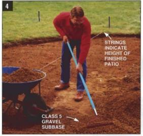
SPREAD CLASS 5 subbase to a depth of 4 in. over entire patio area and 8 in. beyond. Measure down from guide strings to establish uniform height of subbase.
