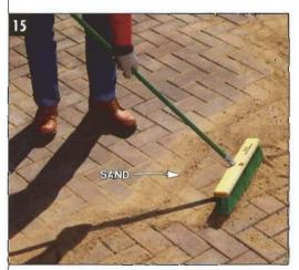
SWEEP COARSE, DRY SAND between cracks of pavers to lock them together and fill voids. Repeat with more dry sand in a few days.
