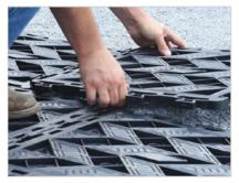
5. Lay *EASYClickBase* on the screeded bedding layer starting at the least difficult point, making sure to stagger joints. Extend 6" beyond pavers.
