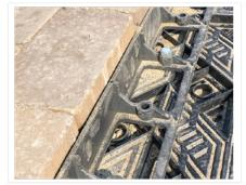
8. Install Snap Edge Paver Restraint or Stronghold Aluminum Edge to properly secure install into place. A fibre reinforced concrete edge such as EdgeCrete can also be used.
