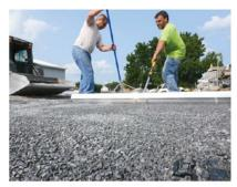
4. Screed #9 stone or sharp sand to ensure compacted level bedding layer is completely flat with no low spots.
