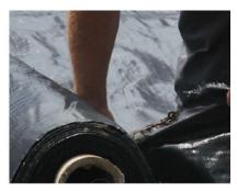
3. Cover surface with non-woven geotextile fabric. Suggested permeability rate of 135 gallons/minute/foot.
