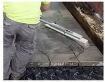
9. Finally, fill all joints with PolySweep or Evolution polymeric sand on driveways, and *EASYJoint* or polymeric sand on all other parts of installation.
