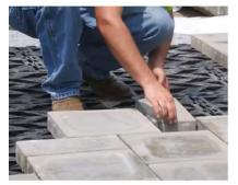
7. Install pavers using standard installation practices. Thin paving materials such as porcelain should be glued to *EASYClickBase* using adhesive such as Paver Bond or BL Platinum.
