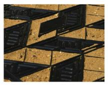
6. For driveways and to increase the load transfer even more, the cavities in the *EASYClickBase* can be filled with bedding layer material. This also prevents waste of any joint fillers.
