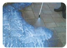
**STEP 1:** Flood coat sealer on surface with a lowpressure sprayer.
